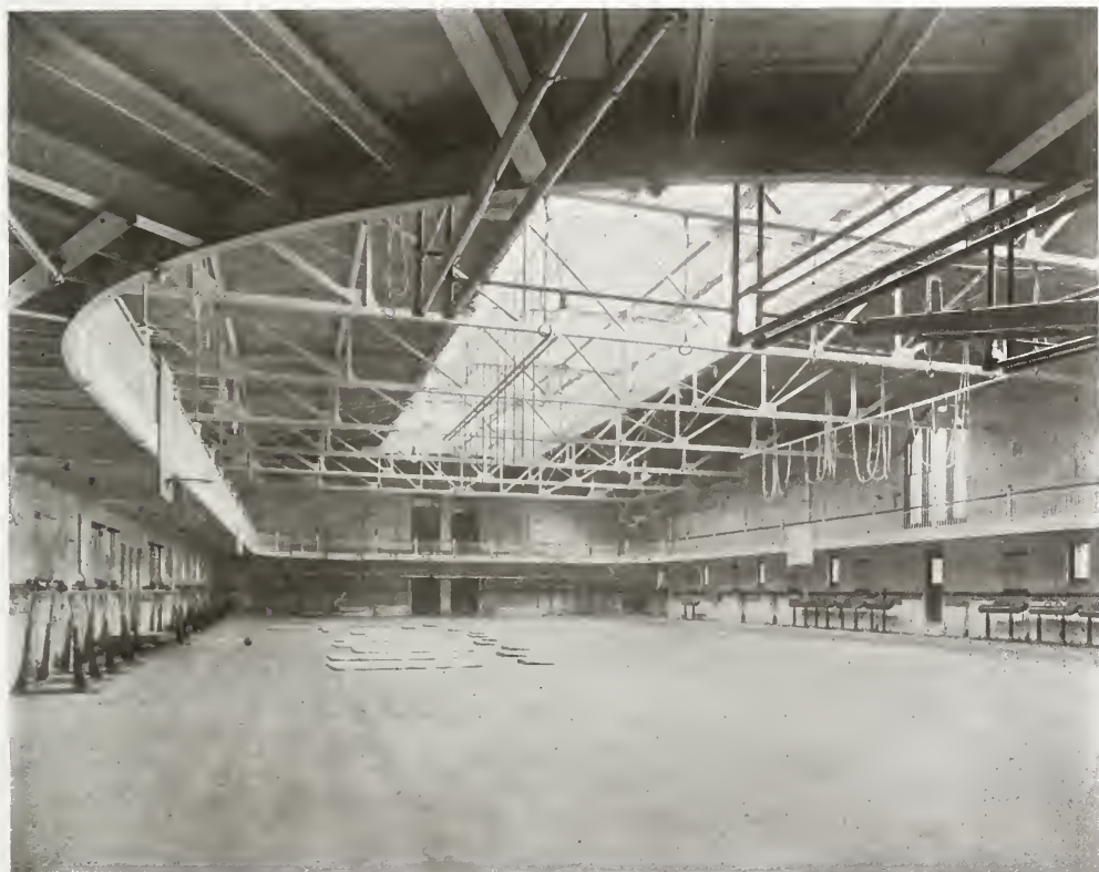
GYMNASIUM—U. S. MILITARY ACADEMY, WEST POINT, N. Y. Cram, Goodhue & Ferguson, Architects, 1908.
